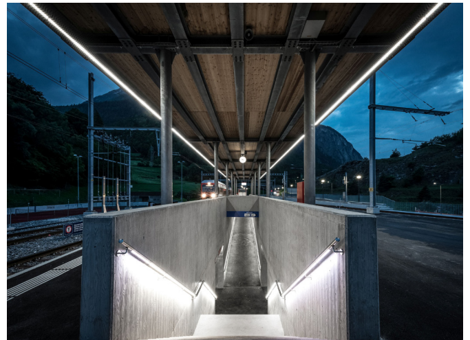
Sembrancher railway station (ceiling: LaneLED WALL, staircase: LaneLED INOX42)
